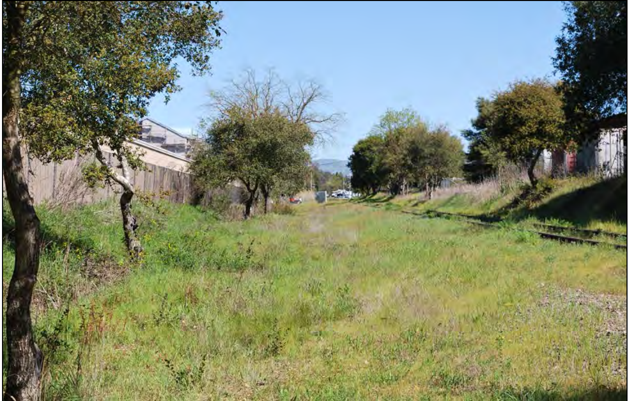
Figure 11: Segment 7 - view north from ca. 900 feet south of Dry Creek Road
