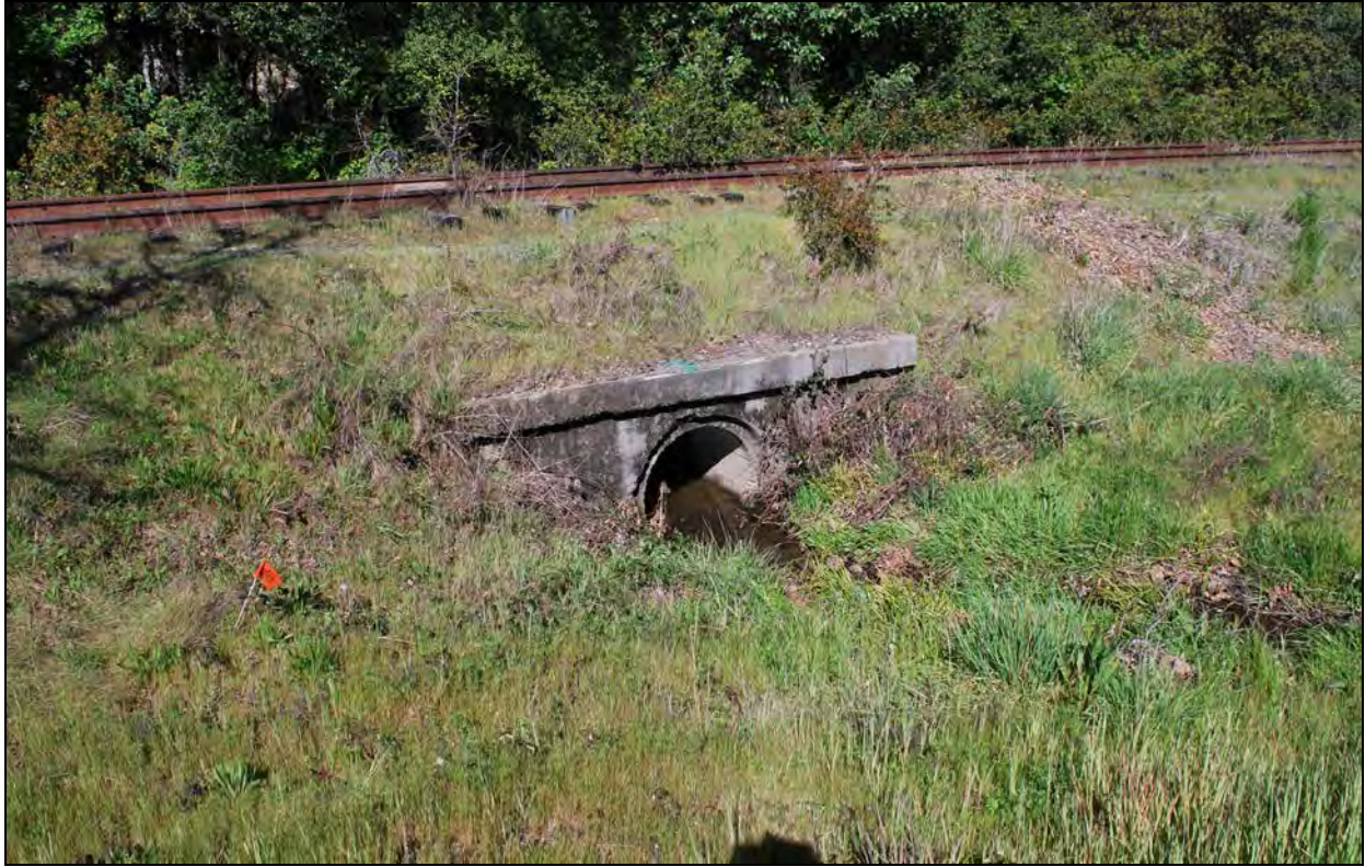
Figure 6: Segment 8 - culvert west of Healdsburg Community Center playground - view west
