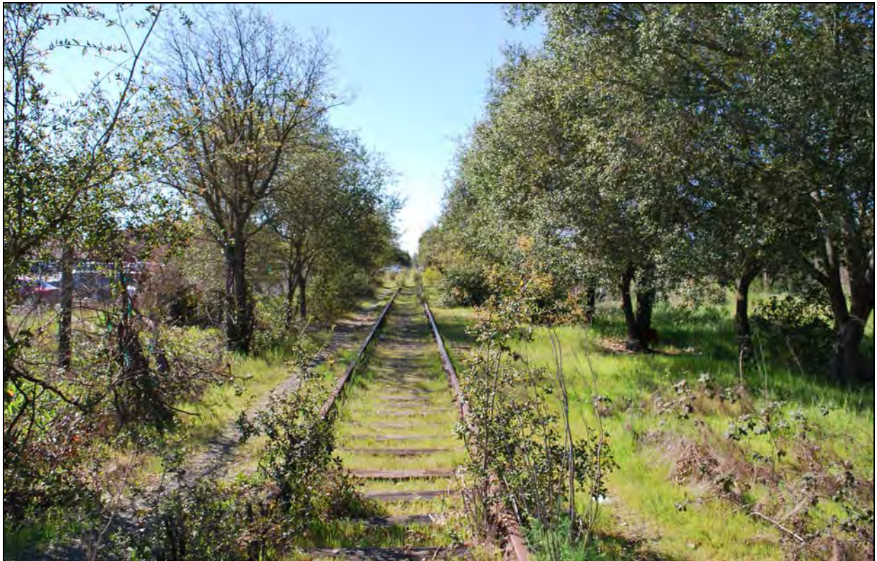
Figure 9: Segment 8 - view south towards Dry Creek Road
