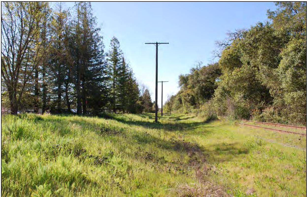
Figure 5: Segment 8 - view south, west of Healdsburg Community Center parking lot
